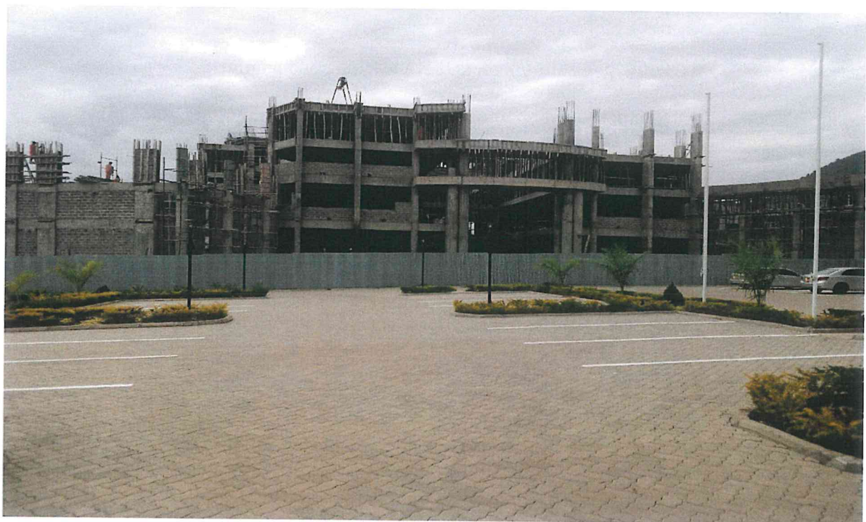
Ongoing Construction of Administration and Lecture Halls Block Phase II
