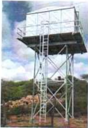
Elevated steel tank for Kiambere Mwingi Last Mile Phase II- Kakuya
