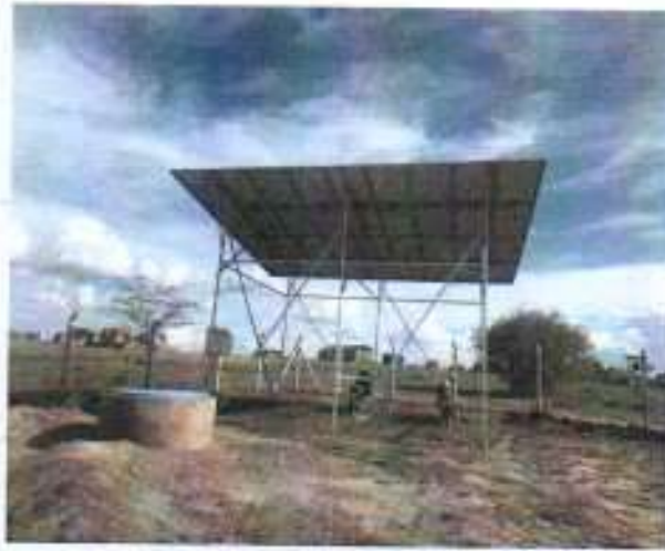
Dr. Likimani primary school borehole enclosed in a bulb wire mesh and solar panels mounted next to it.
