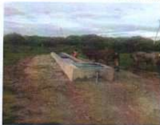
Cattle trough at Kithina Borehole
