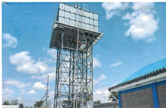
Mavoko Drinking Water Project- Syokimau_300m 3 Elevated tank
