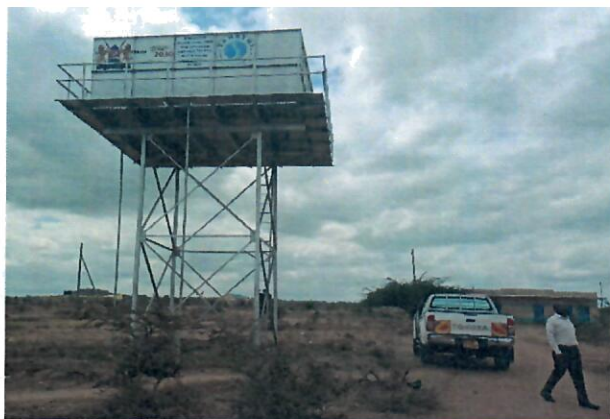
Masinga-Ikaatine-Ekalakala Water Project - Elevated tank at Kanyonyo market centre
