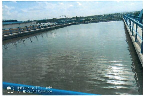
Mavoko Drinking Water Project Water Treatment Plant- Pre-settlement Tank
