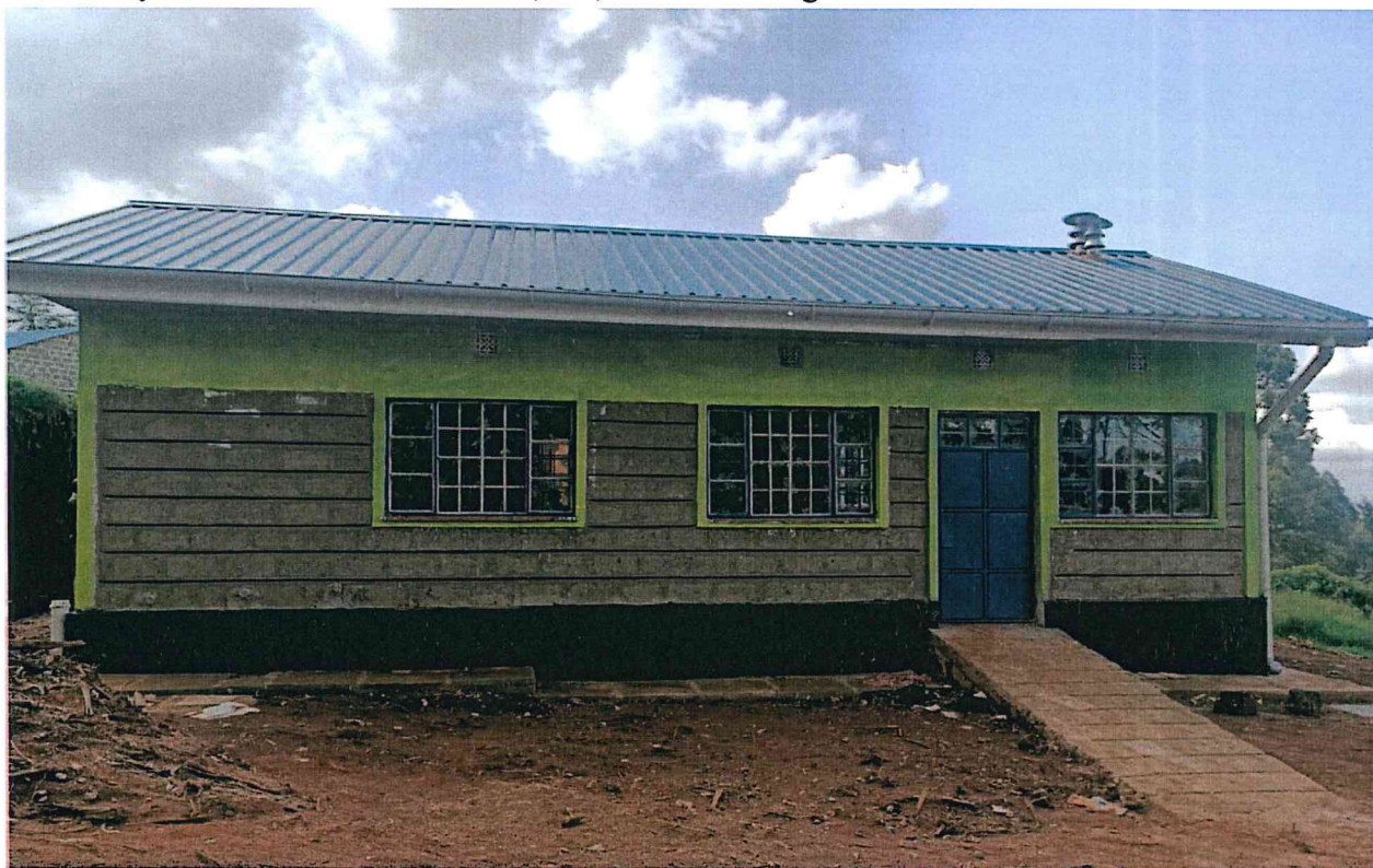
Figure 12: Completed kitchen for Kabebero Mixed Secondary School
