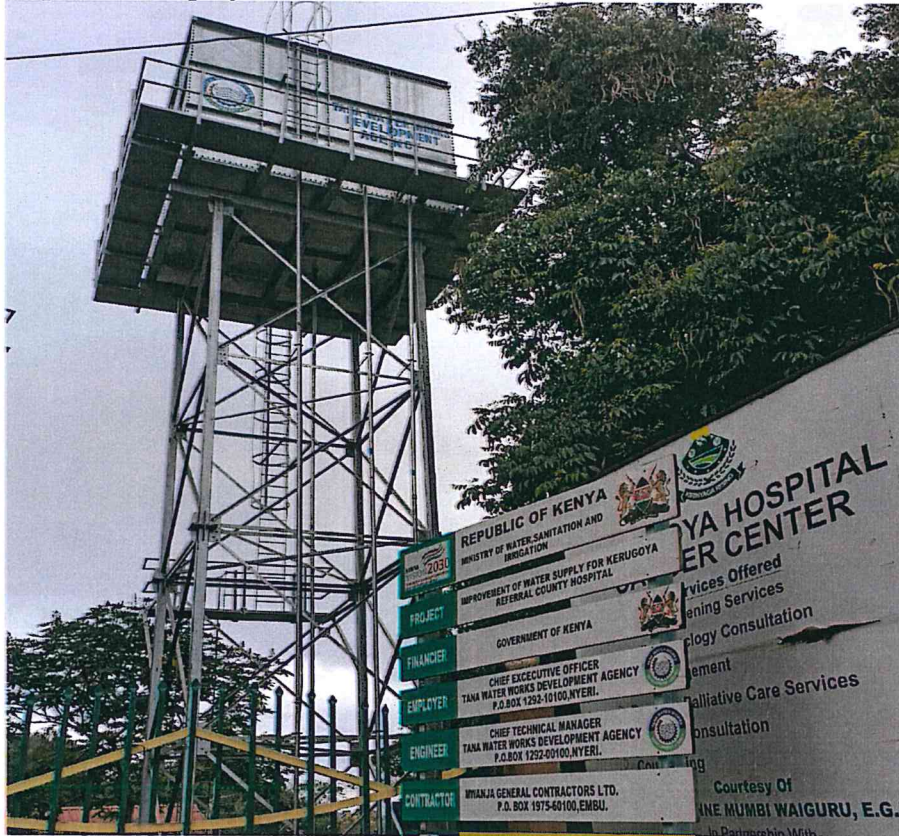
Figure 4: 48M3 steel Elevated tank at Kerugoya Referral Hospital
