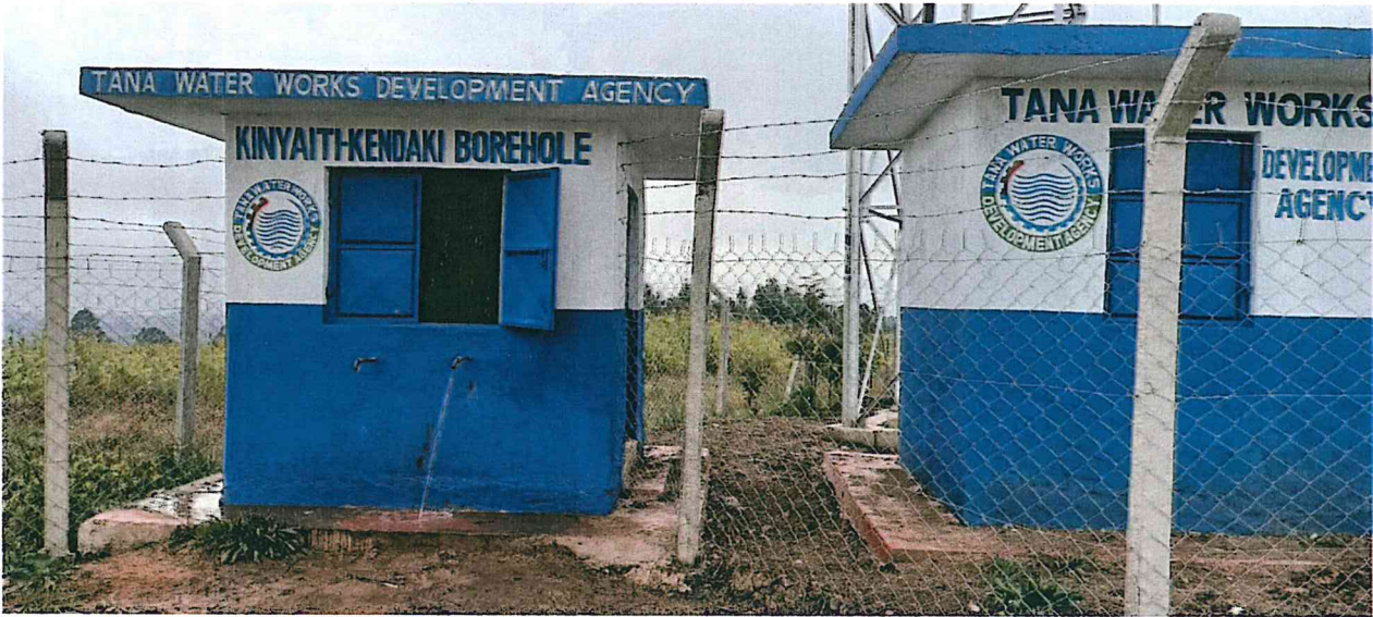
Figure 6: Pump house and water Kiosk at Kinyaiti-Kedaki Borehole with a yield of 54m 3 /day in Kieni, Nyeri County
