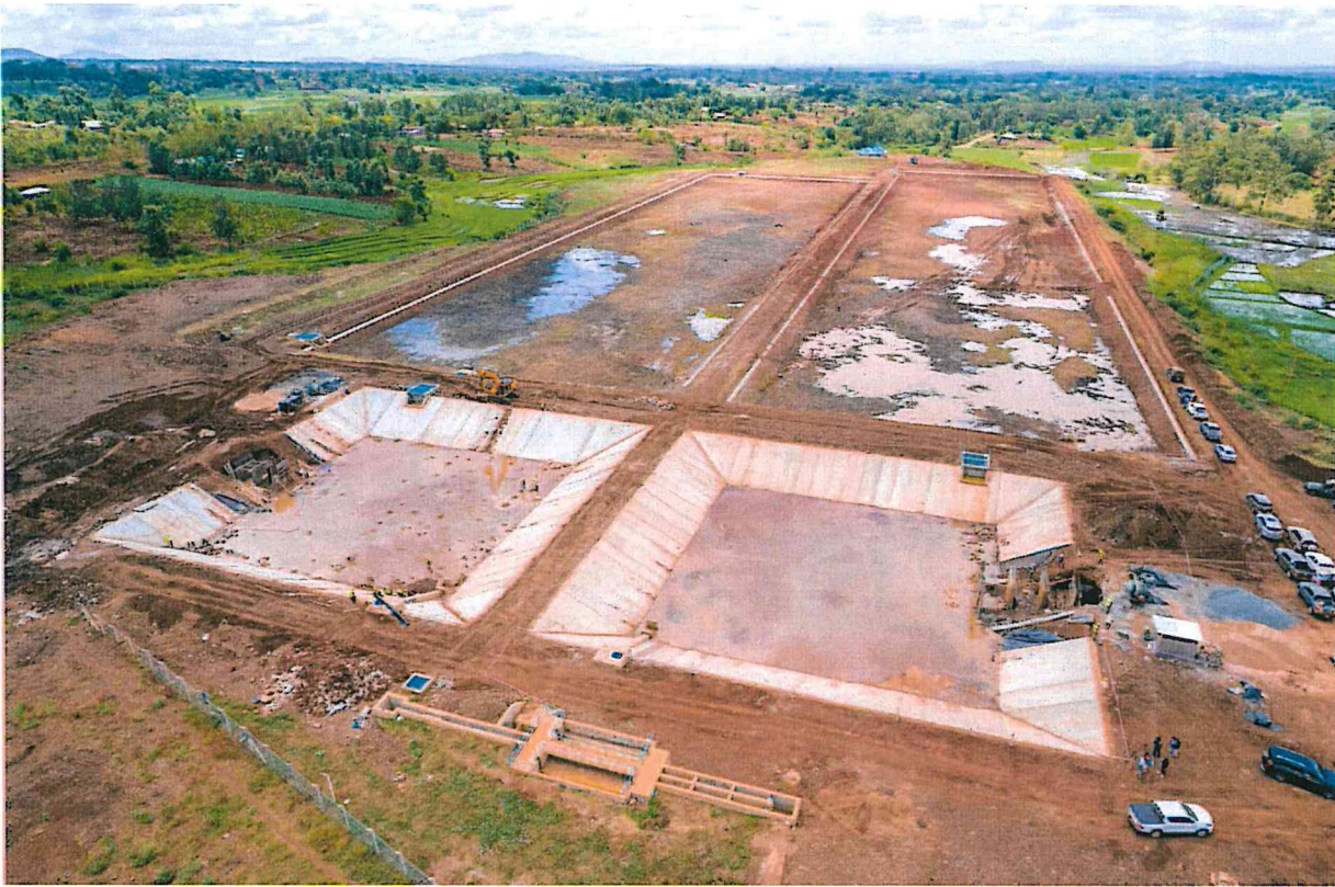
Figure 1: Rwanyange sewerage treatment plant at Meru Sewerage Infrastructure. The sewerage treatment capacity is 8,000M 3 per day.
