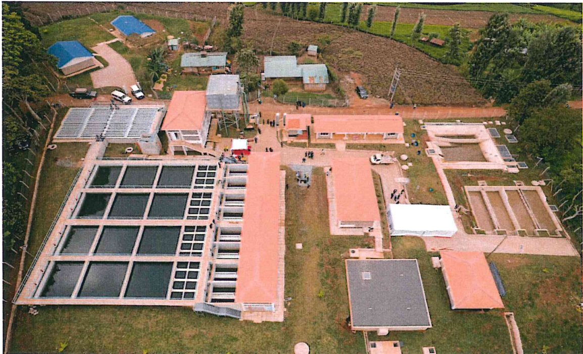
Figure 3: Completed Treatment Plant at Chogoria Water Infrastructure
