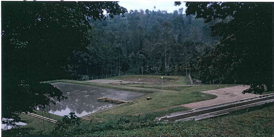
Figure 5: Completed Othaya Sewerage Project - Last Mile Connectivity
