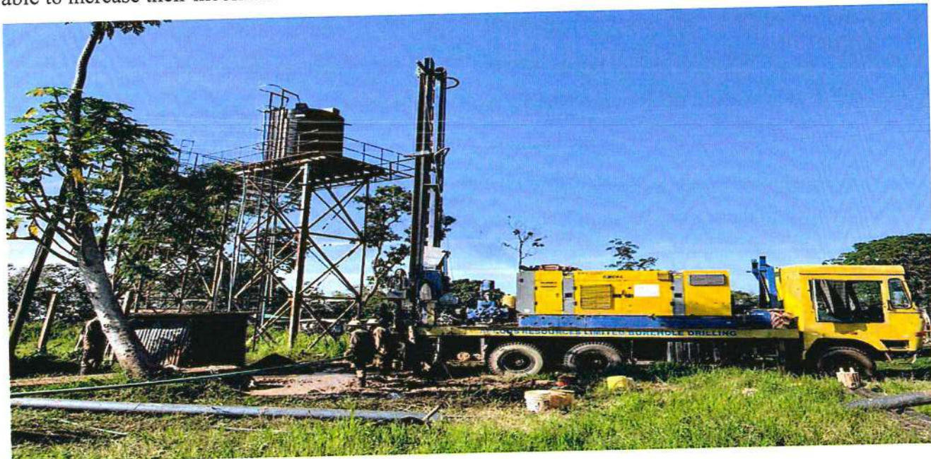
Drilling of a borehole
