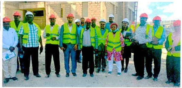
NHC Board members and the technical team during inspection of the Stani Athi Sector 2A. The units will be ready for occupation by July, 2024.
