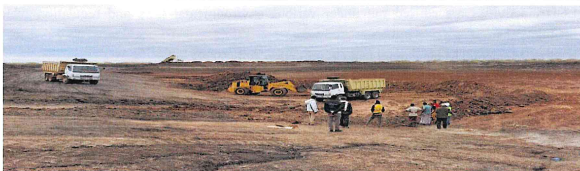
Photo 1. Community members observe the excavation works.
