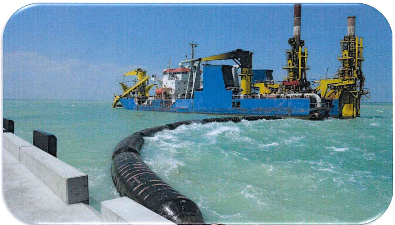
Figure 2: Dredging channels at the Port of Lamu
