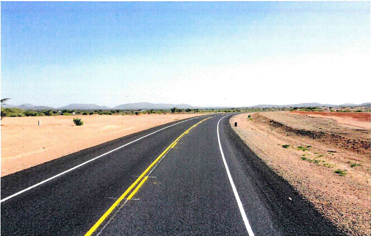
A section of the Lokichar-Lodwar-Nakodoko 330 Km Highway
