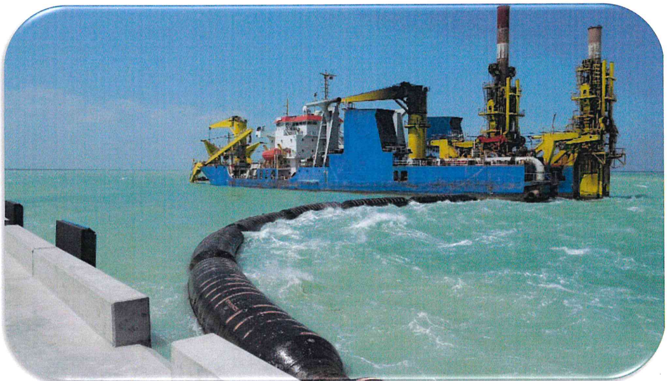
Figure 2: Dredging channels at the Port of Lamu
