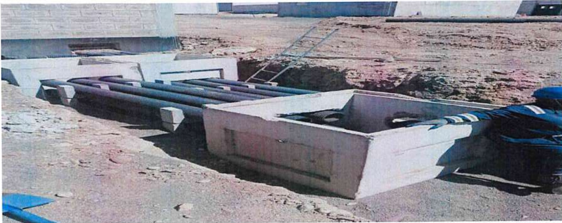
Laying of LV Network at the Water Treatment Plant
