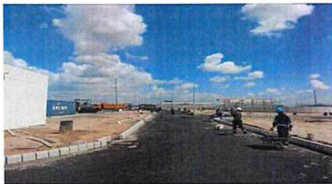
Installation of road kerbs at the WRF road network.
