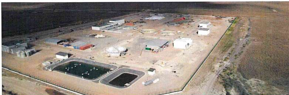
Ariel view of the Wastewater Reclamation Facility
