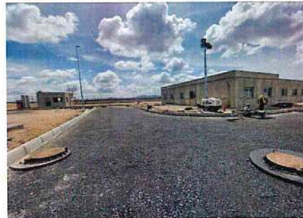
Priming of road surface at WRF roads
