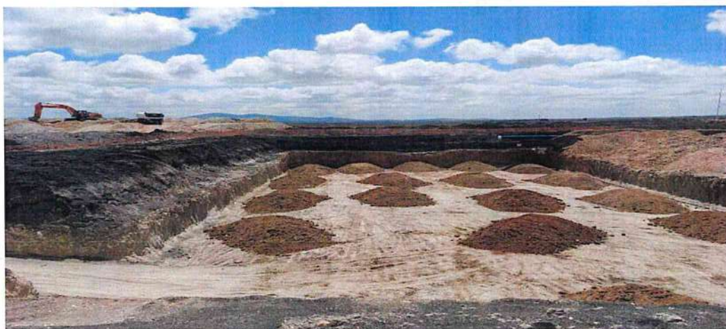
Backfilling at the Solid Waste Sorting Facility.
