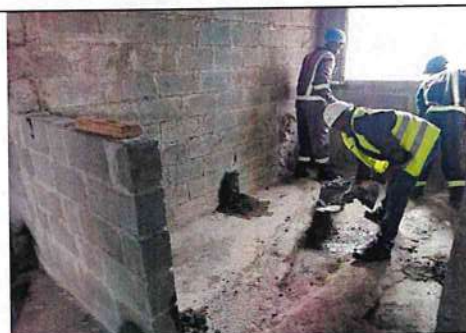
Setting of levels at WTP Maintenance Building
