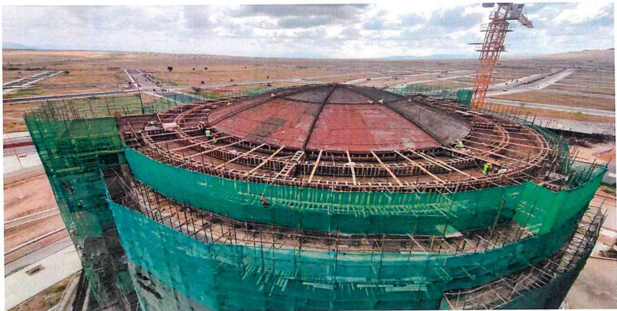
5 th Floor – Dome and roof gutter beams and slabs
