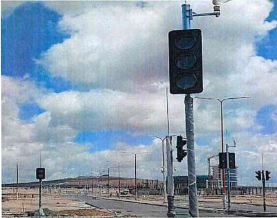
Traffic light poles installed in the city.
