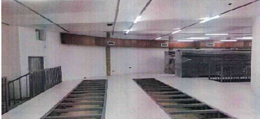
Construction of Data Centre Disaster Recovery Centre
