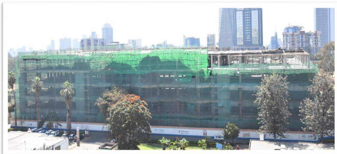
Burns Management and Paediatric Emergency Centre under construction
