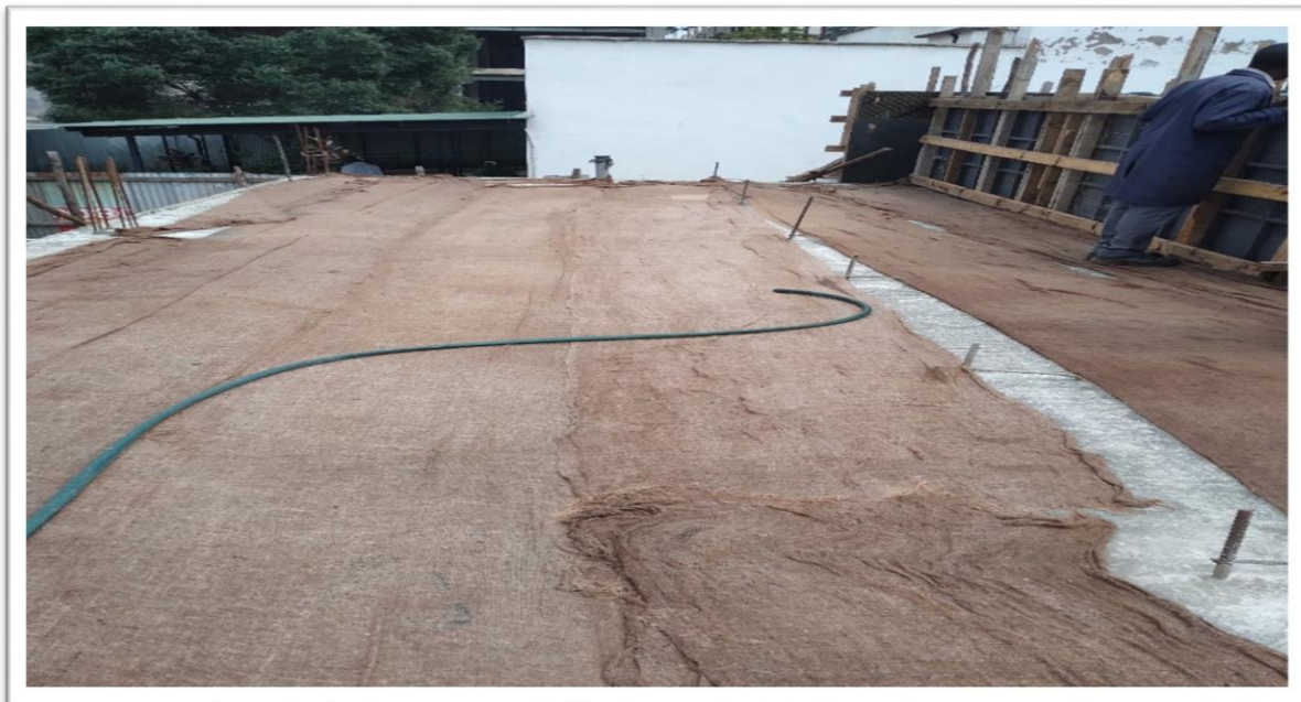
Construction of Bunker at 80% complete
