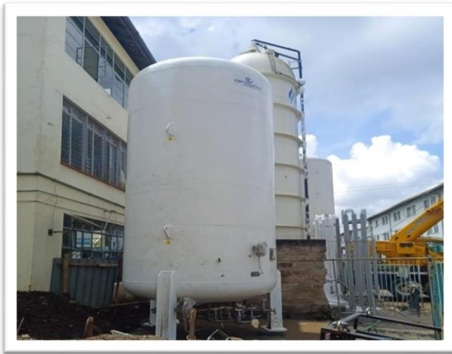
Oxygen tank installation
