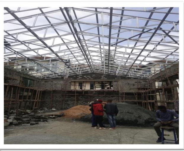
Oxygen plant housing under construction
