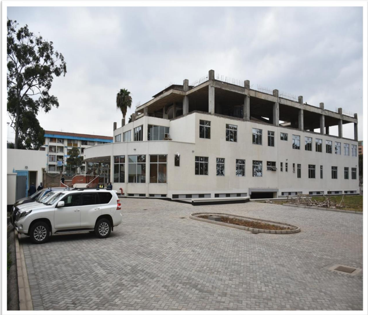
Construction of Cancer Center phase I at 100% Completion
