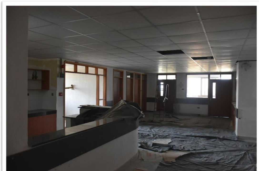
Tower Block 8 th Floor renovation at 45% completion
