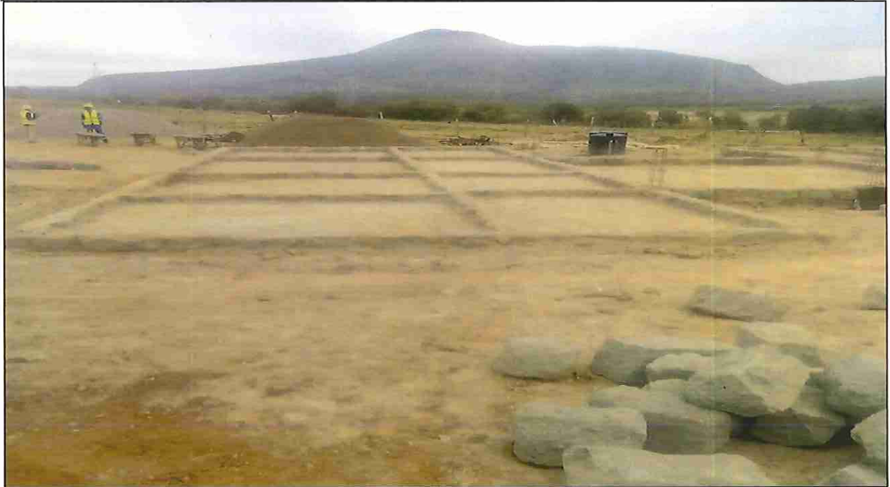
Narasha dispensary at foundational stage
