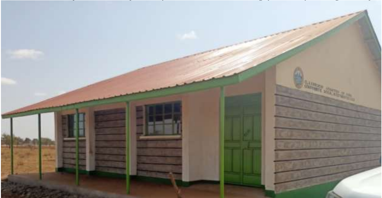
Construction of a classroom for Mbukani Primary School in Machakos County.
