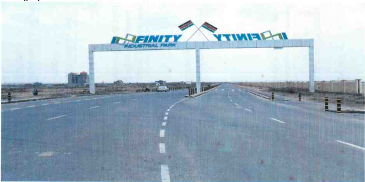
Figure 6: Completed section of Infinity park roads
