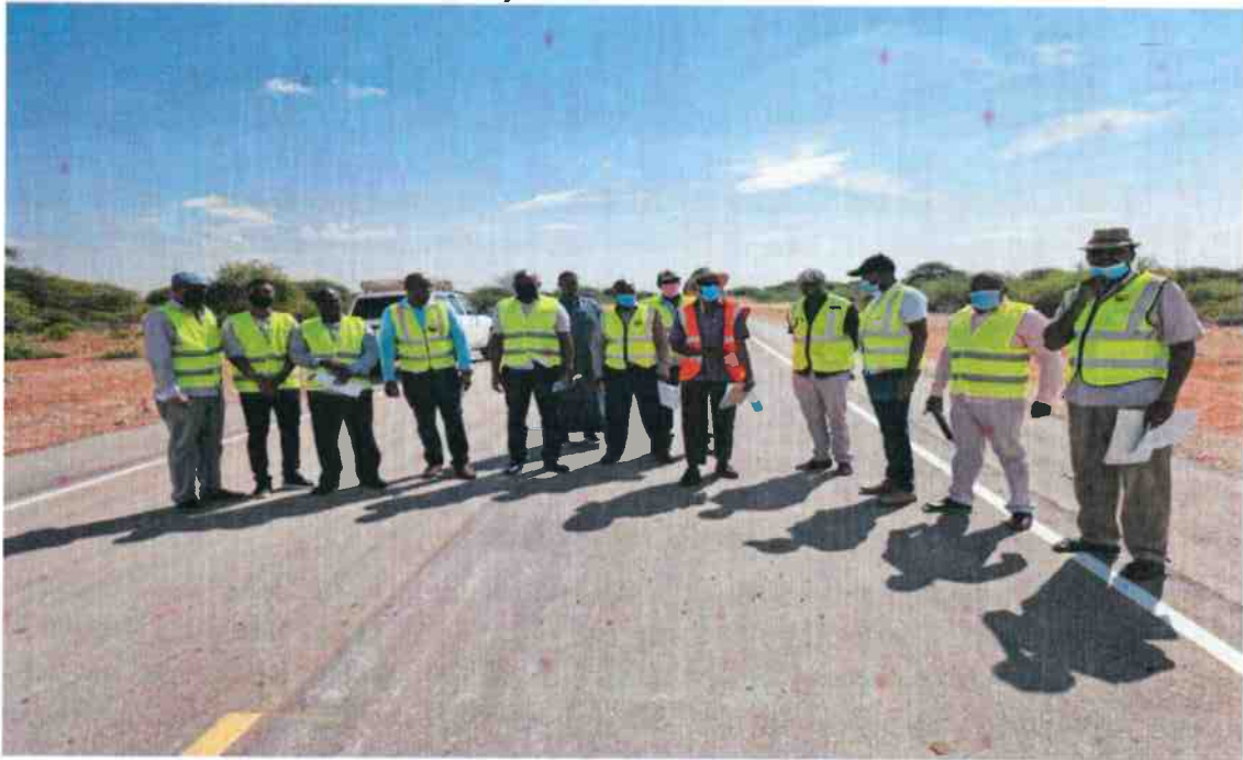
Figure 13: Quality Control - Inspection of works during substantial inspection of the upgrading of 8km Wajir bypass phase 1
