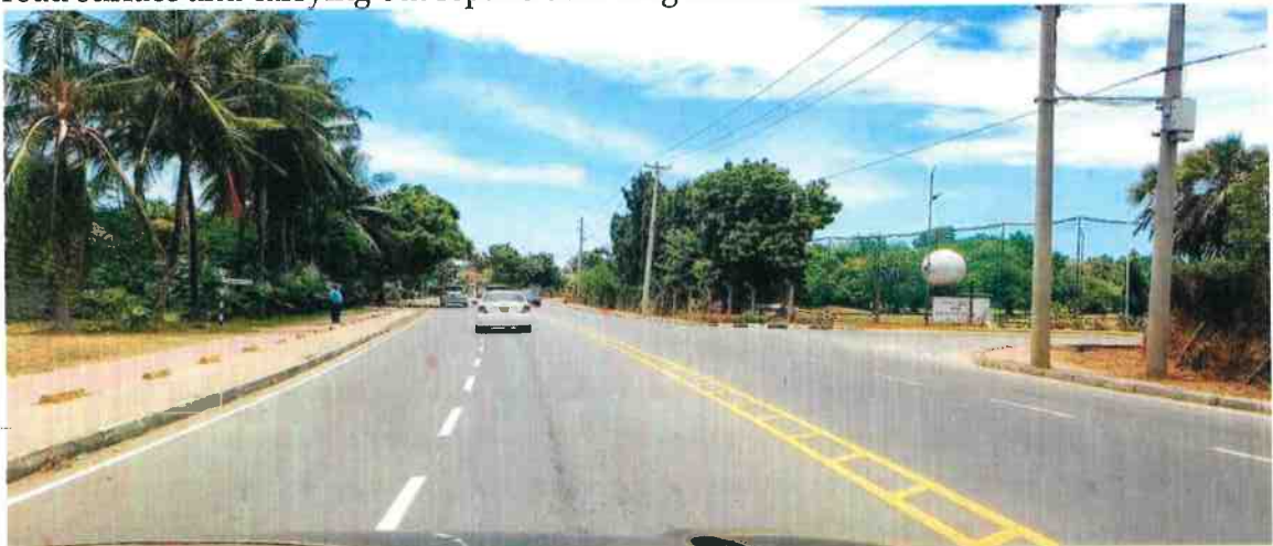
Figure 10: Rehabilitation of Links Road Nyali, Mombasa County
