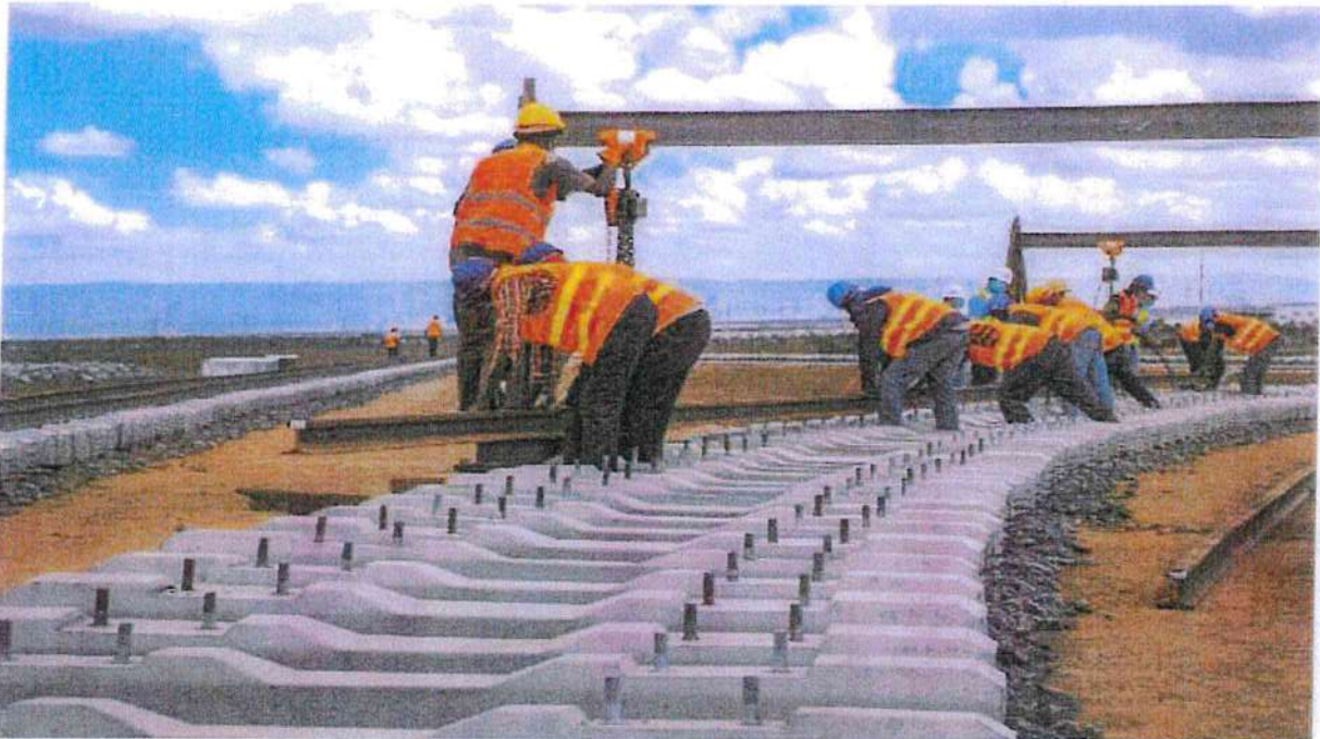
Construction of Naivasha - Longonot
