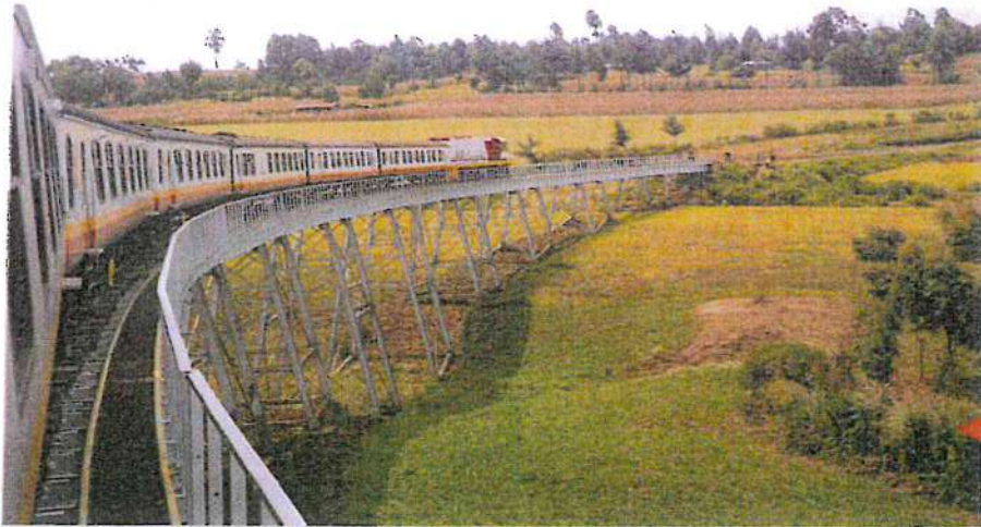
Nanyuki bound passenger train navigating over one of the rehabilitated bridges. Nanyuki boasts of its scenic landscapes and the magnificent Mt. Kenya, which is a favourite spot for hikers. Since the rehabilitation of the Nairobi- Nanyuki railway line, we have transported over 45,000 passengers to Nanyuki.
