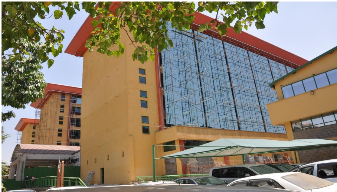
The New Mitihani House (Ongoing Project)
