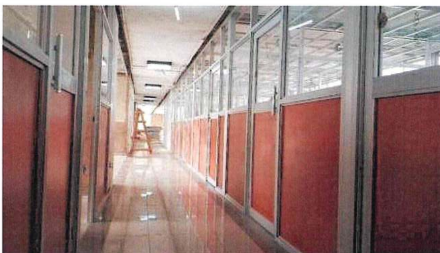
Ongoing office renovations at the 14 th floor (KNATCOM offices)
