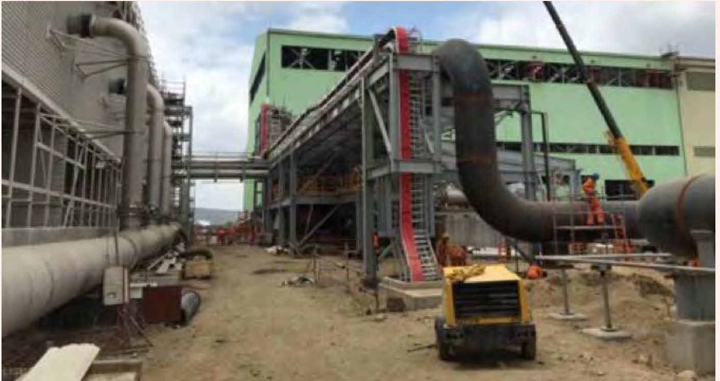
Olkaria I Unit 6 power plant construction in progress
