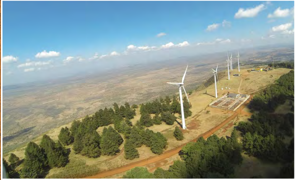
Ngong Wind Farm
