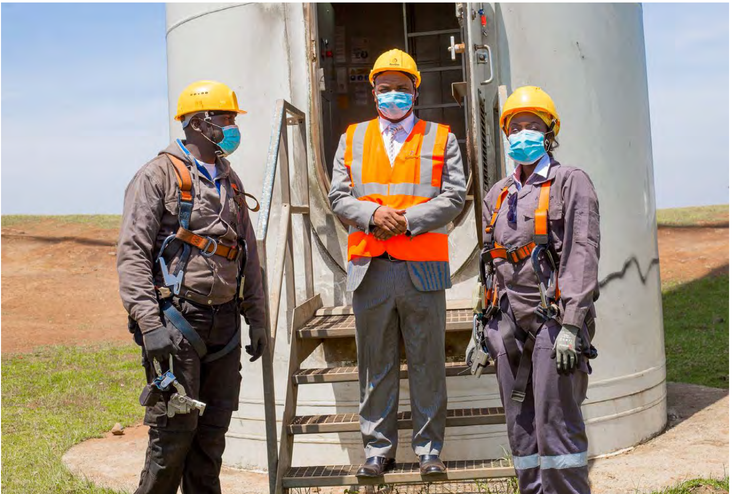
KenGen engineers preparing to climb one of the Ngong Wind Masts for a routine maintenance job
