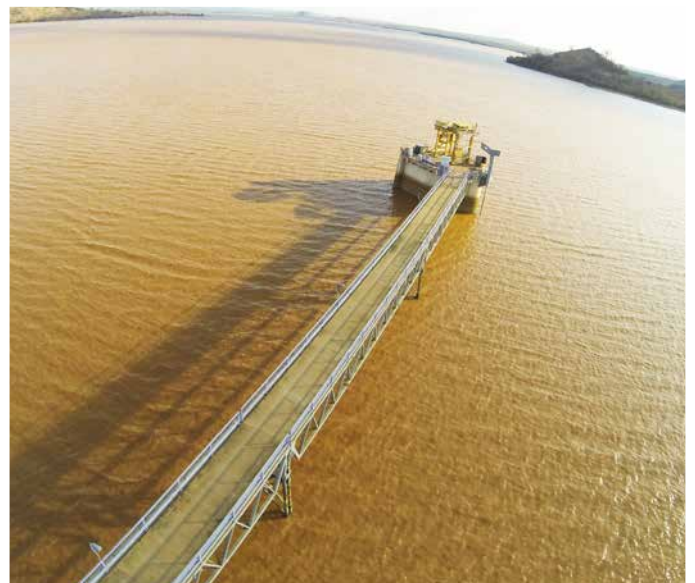
Largest Hydro-powerplant Kiambere 168MW in 2009
