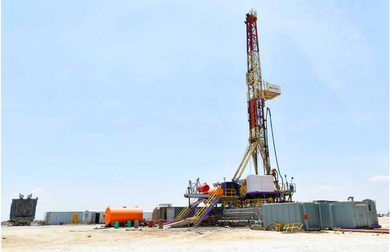
KenGen Geothermal Rig
