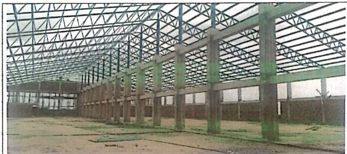
Steel structure ready for roofing.
