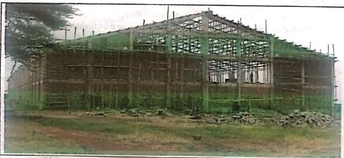
Oloitokitok Agro-Processing project super structure under construction
