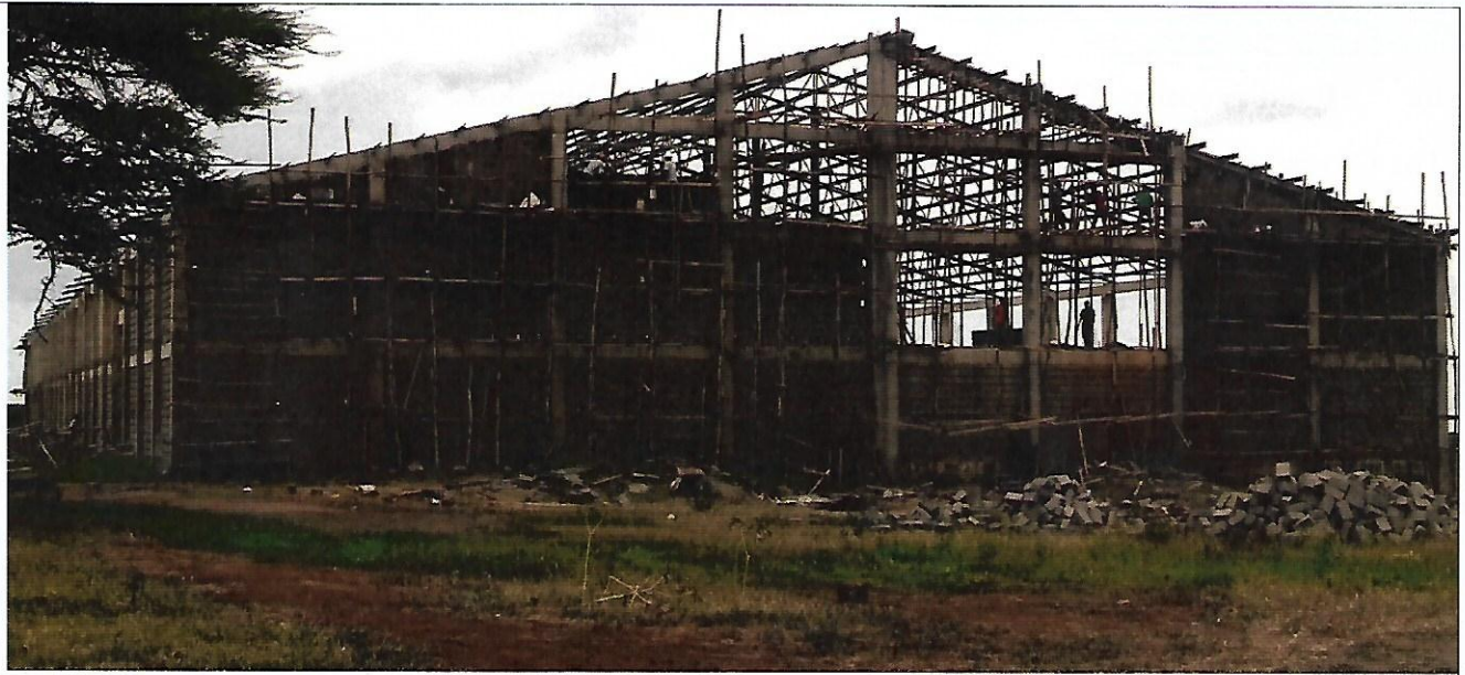
Oloitokitok Agro-Processing project super structure under construction
