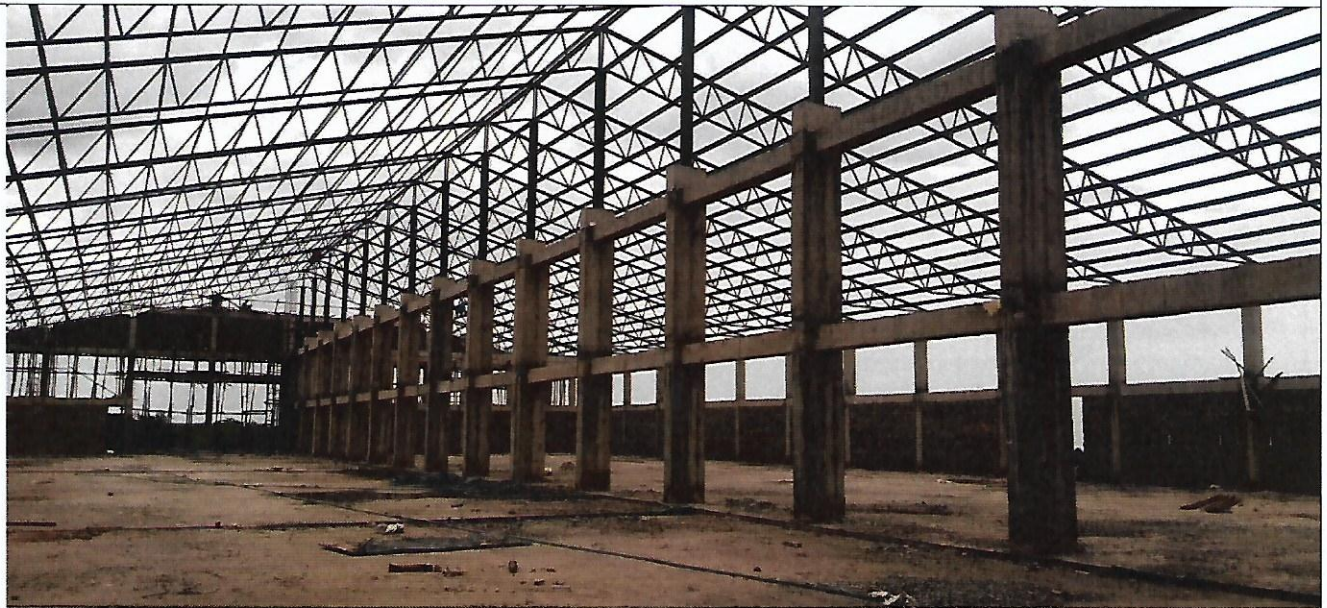
Steel structure erection in preparation for roofing.
