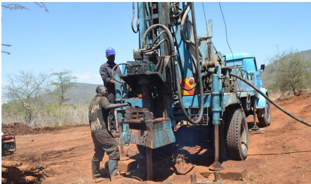
Borehole sinking in Kajiado to combat drought.
