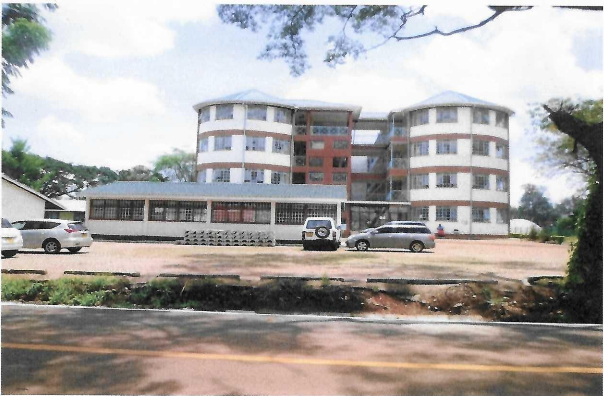
Figure 8: College internal Access roads
