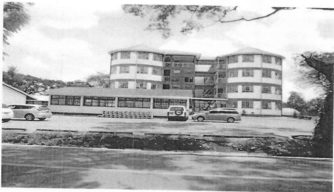
Figure 8: College internal Access roads
