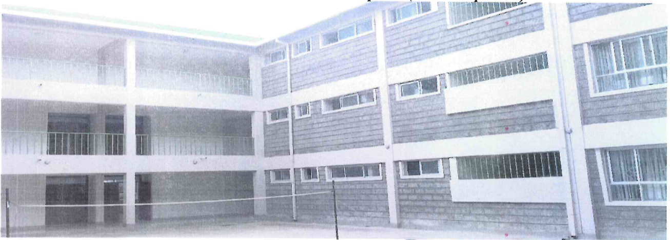
Picture 3: Library Block Under Construction (Front Elevation)- 55% completion
