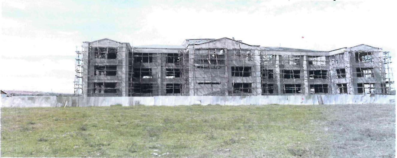
Pictures 4: Students Multipurpose Hall under construction- 90% completion
