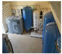
To meet the rising demand for CCU, Mwai Kibaki Hospital constructed and operationalized an Oxygen plant with a capacity to produce 1,500 litres of oxygen per minute, 2,160,000 in 24 hours, and has 18 ports filling station with an ability to fill in 72 oxygen cylinders in 24 hours. The Hospital also acquired a 3000-litres bulk liquid oxygen tank in the FY 2021/22. The facility is supporting the provision of oxygen to other health facilities within the region.
