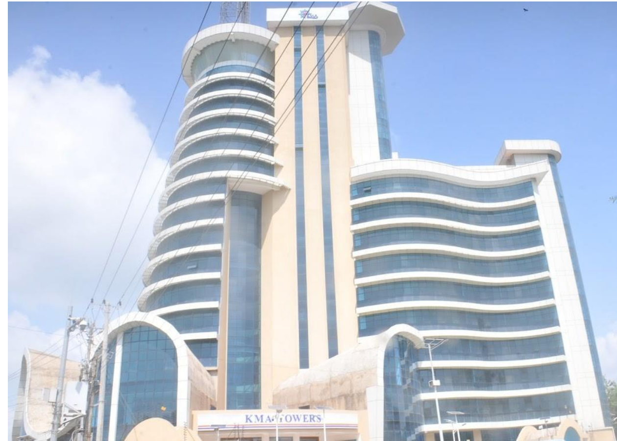
Kenya Maritime Authority Headquarters
