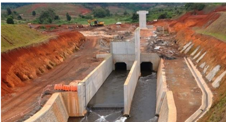
Construction of Thiba Dam
