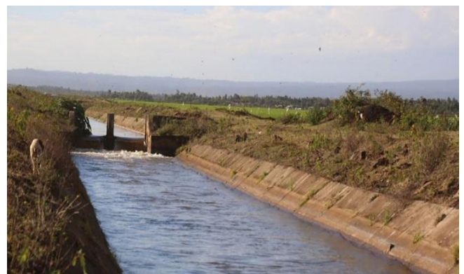
Rehabilitated water pan
