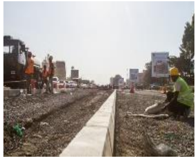
Ongoing road construction in Ruaraka Outer ring road
