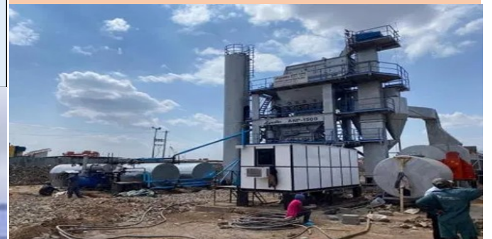
Asphalt Plant Constructed in Kangundo by NMS used for processing bitumen and asphalt
