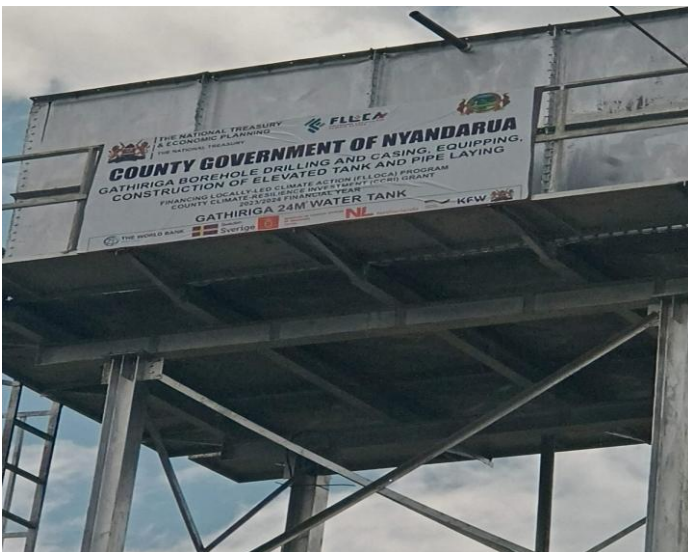
Figure 11: Githiriga water project in Nyandarua County was completed and has been commissioned at a cost of 11.5 M. The County bought land while FLLoCA funded drilling of borehole yielding 25M3 per hr, installation of 34 solar panels 545 Wtz, installation of an elevated tank of 75M3, piping and renovation of an existing community water tank of 50M3
