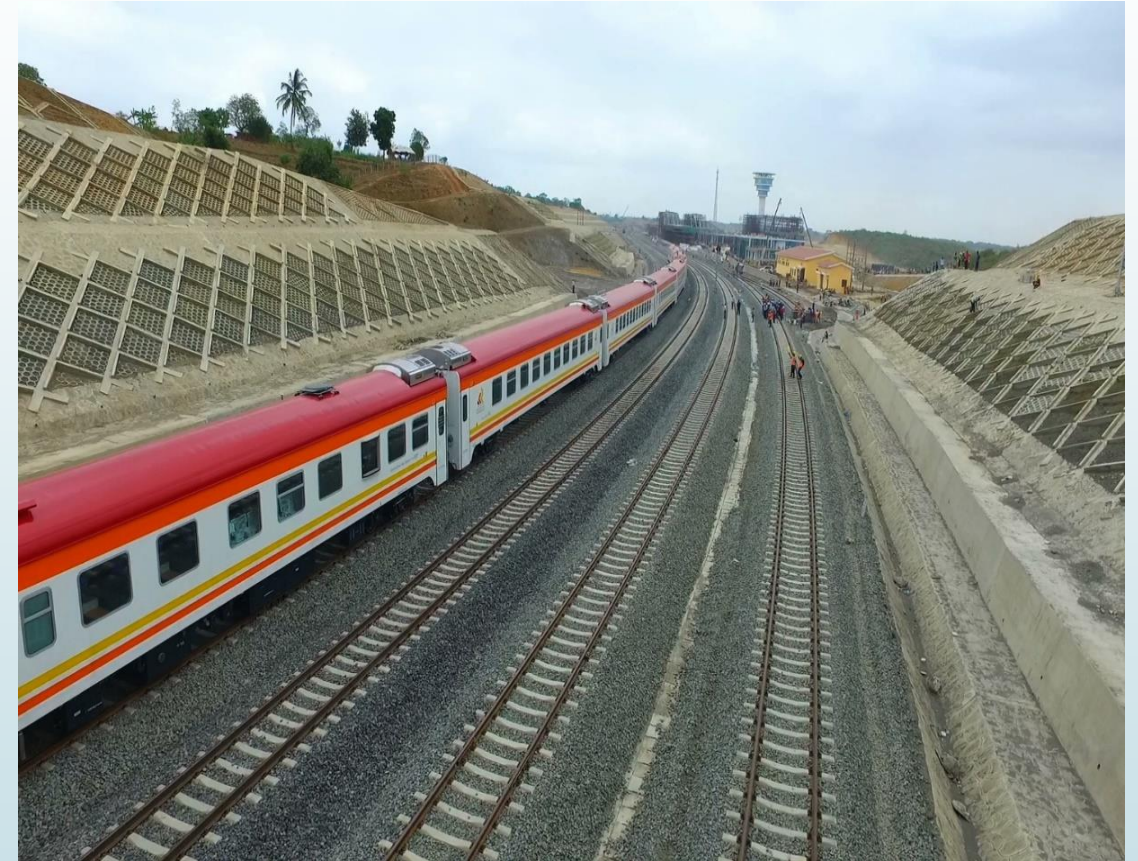
Improved Passenger and Cargo Handling (Nairobi-Mombasa SGR)
