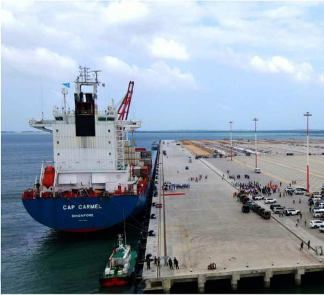
Improved Domestic and Regional Trade (LAPSSET Corridor - Lamu Port)
