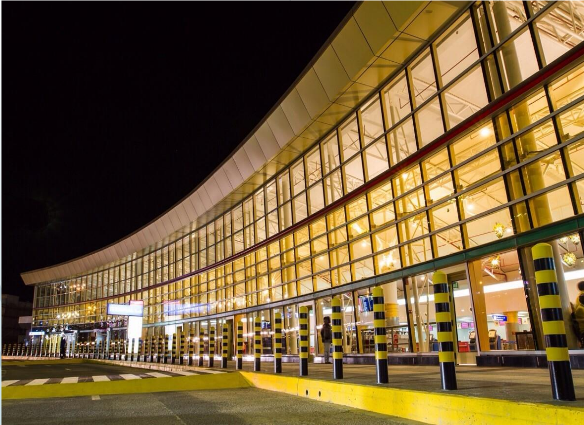
Increased International and Domestic Passenger Handling (Modernization of JKIA)
